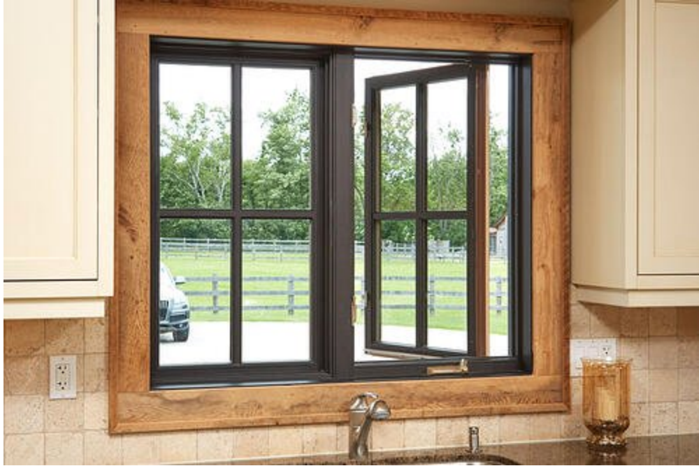
Type A: hinged on the side, and cranks or swings outward
